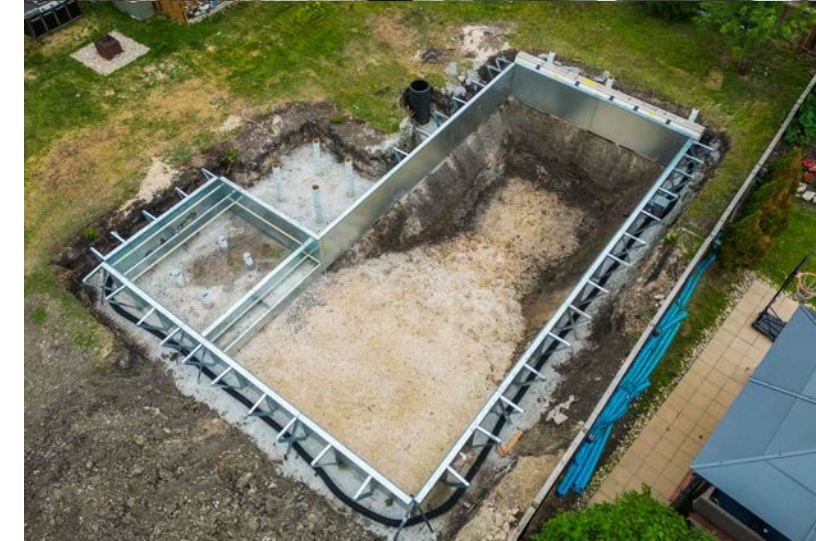
Aerial view of a 16' x 36' rectangle steel kit with 42" G235 steel panels, with an added 10' x 10' sun ledge/stair combo.
