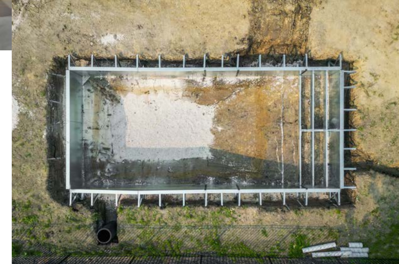
Birds-eye view of a 14' x 28' steel pool kit in construction.
